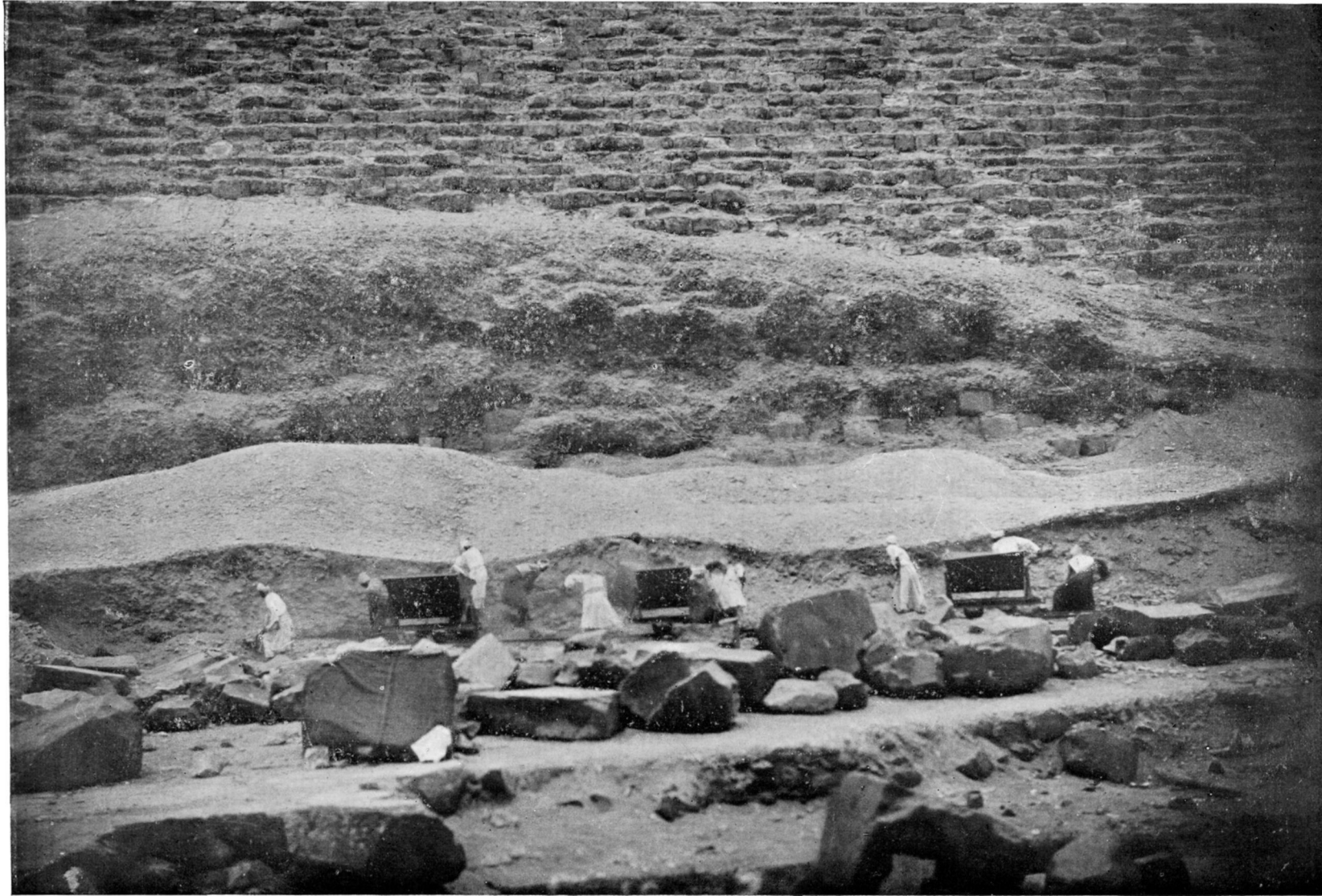
The mound of debris against the eastern face of the Pyramid, and covering the site of the western part of the Mortuary Temple. In the foreground are some of the basalt blocks of the temple pavement
