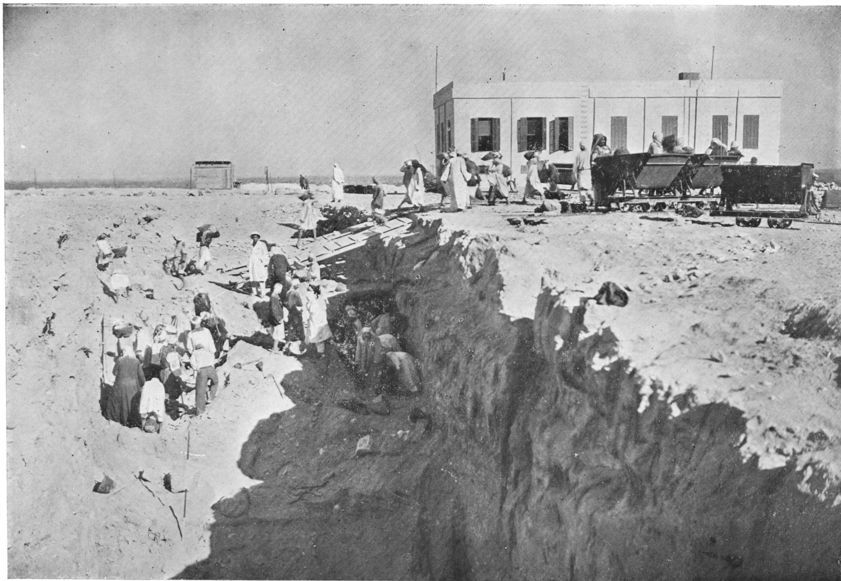
Commencing the clearance of the northern boat of Khufu
